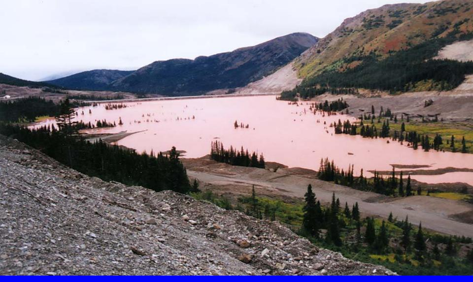
Except for a slight increase in Se, deposition of tailings from oxidized ore has had no adverse impact on impoundment water quality at Kemess.
