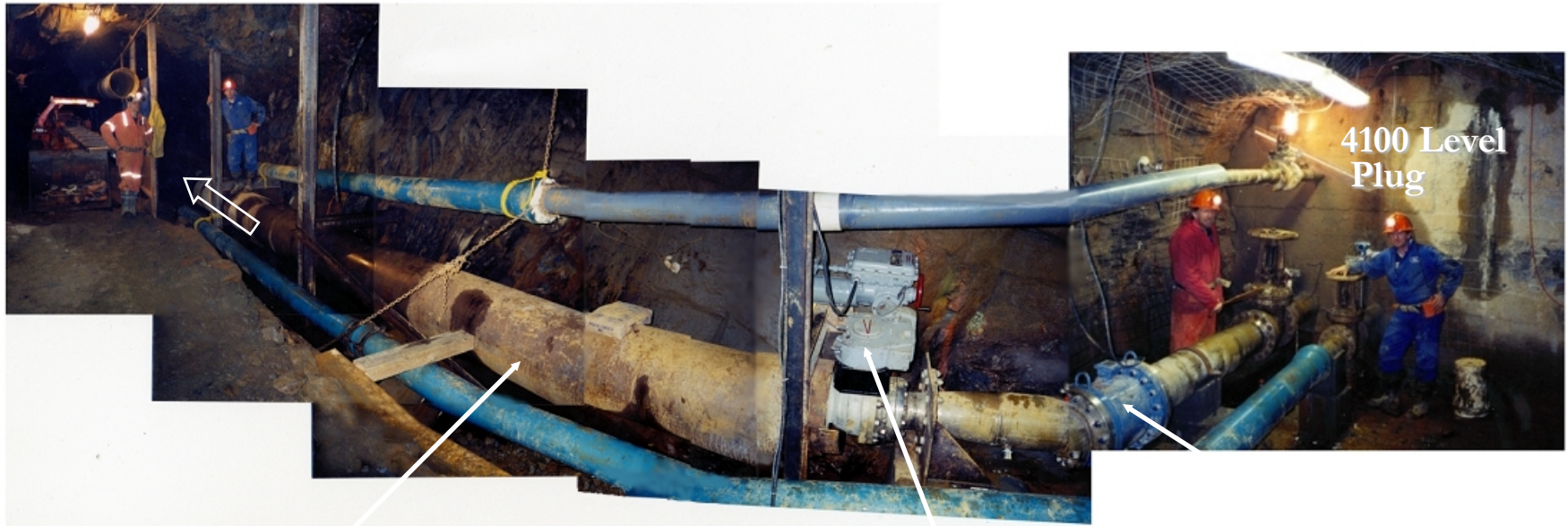
Control Valve and Actuator
