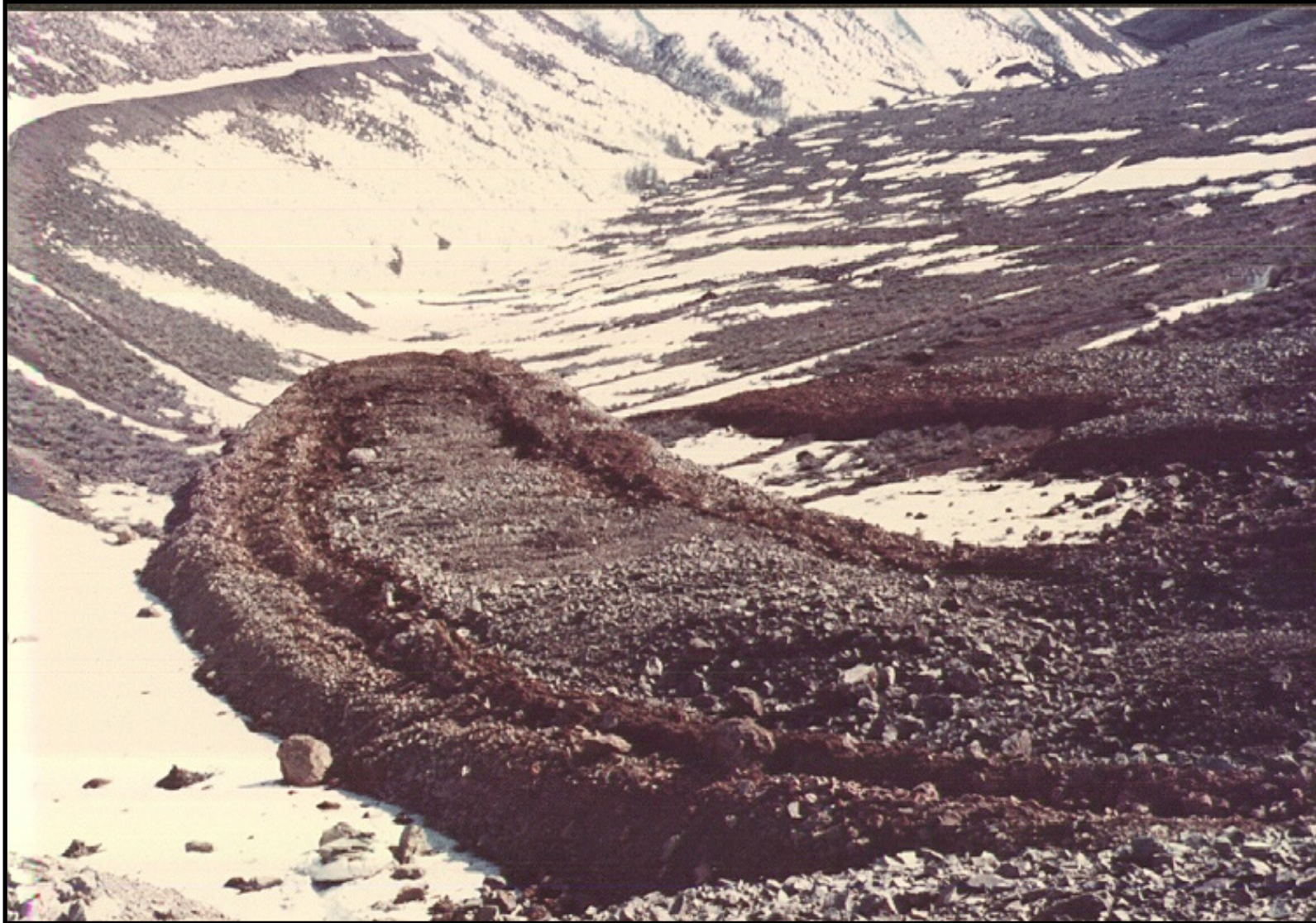
View of run-out tongues showing coarse nature of most mine rock.
