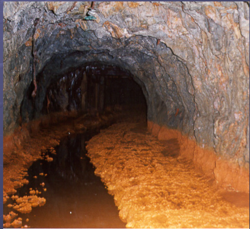
Iron hydroxide sludge, 4150 level
