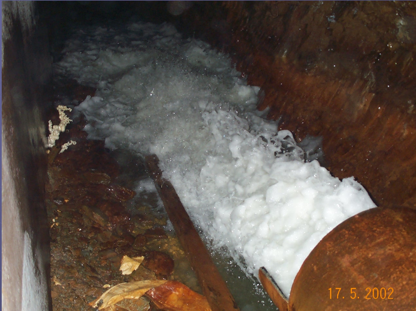
Release of Water During 2002 Plug Test
