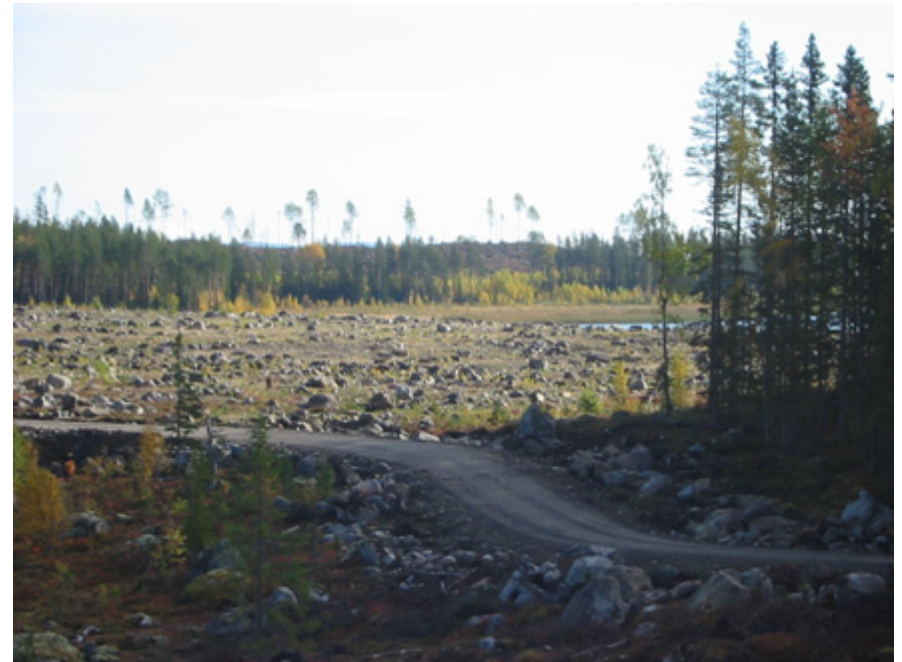
Till covered section of tailings pond
