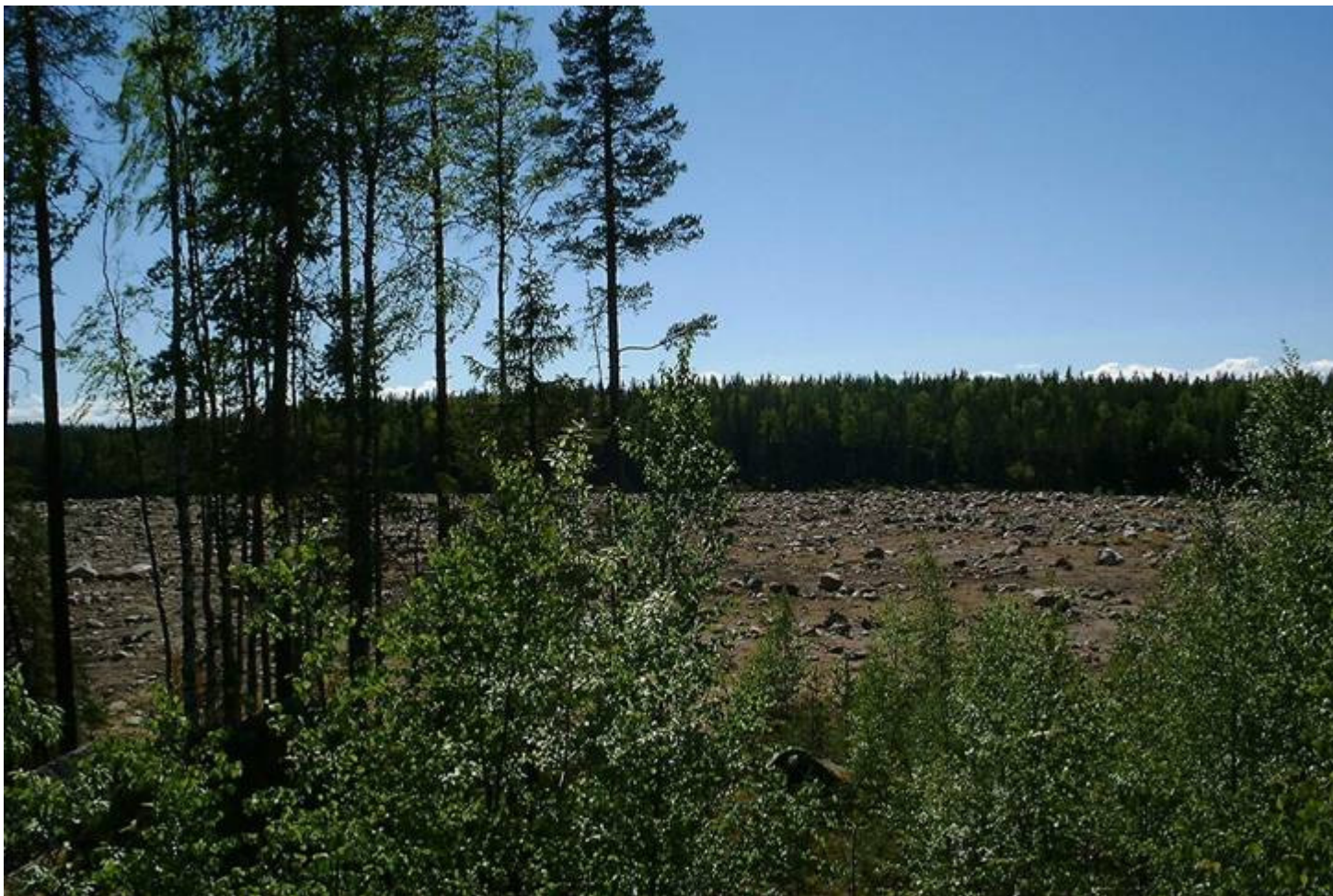
Dry cover section of tailings pond
