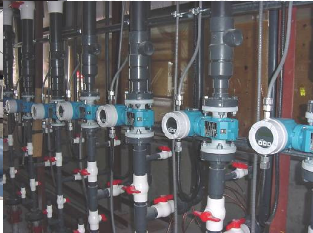
Flow monitoring equipment
