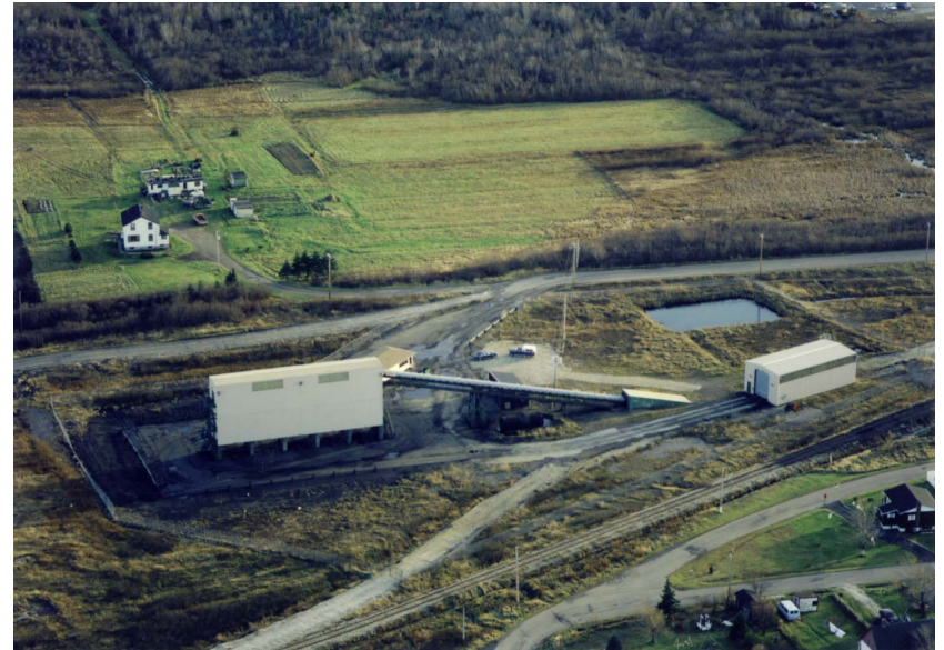
□ Domestic Coal Loadout
