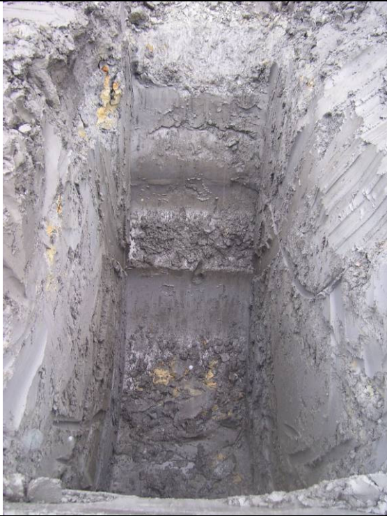
Looking north at the test pit after 3.5 hours. Test pit depth is 6 m. Width is approximately 1.3 m (width of digging bucket).
