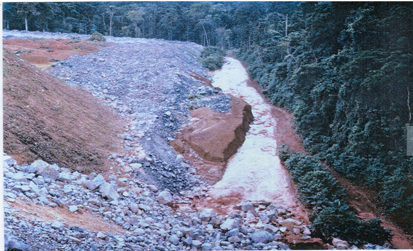
AUGUST 21, 1995 - Seepage flow at toe of north end of the main dam.
