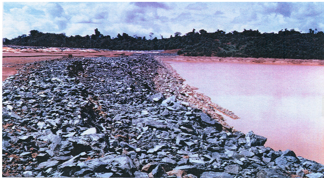
AUGUST 23, 1995 - Upstream face of main dam. Note: Vertical scarps developed above sinkhole thought to be in the original area of failure.
