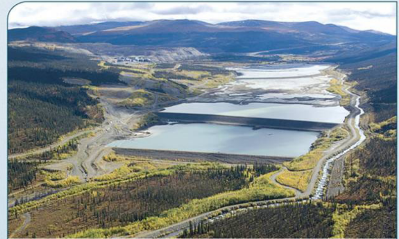
Before remediation (Now)
