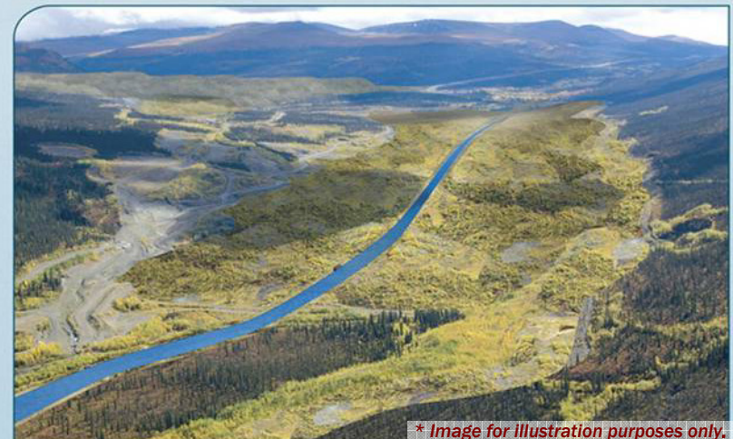
After remediation (approximately 40 years time)
