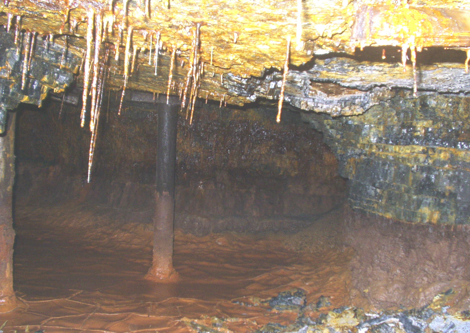
MacKay's Corner "bootleg" workings and AMD formation
