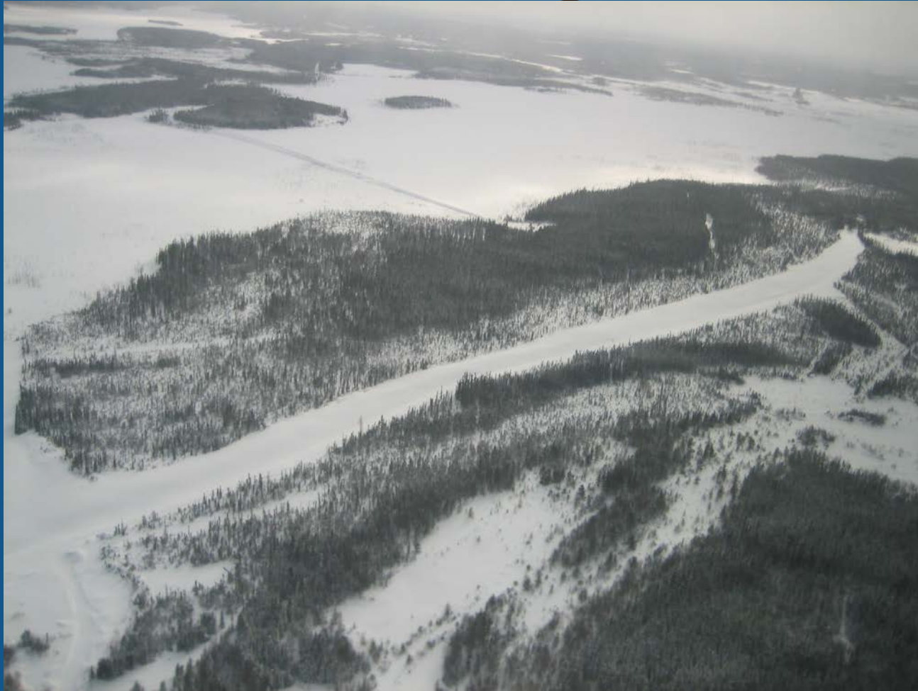
Clean Water Diversion
