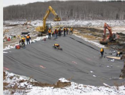
Impermeabilisation of dikes
