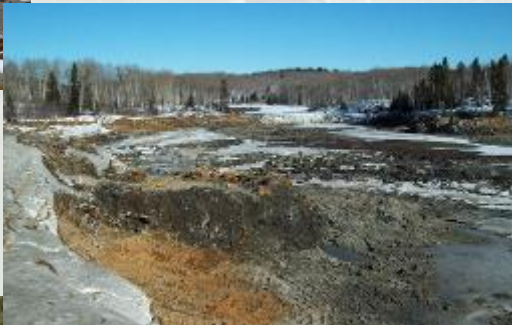
Excavated Intermediate Sector
