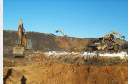
Placement of tailings in a mound
