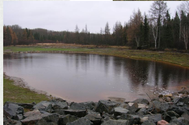
Stream 1 Sector - Settling basin
