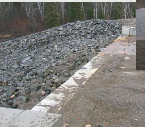
North Sector - Spillway
