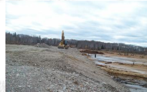
Placement of the monolayer
