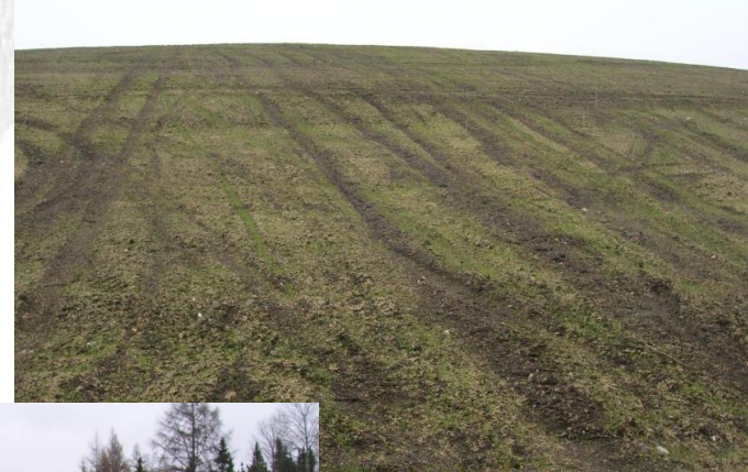
South Sector - Seeded impervious cover
