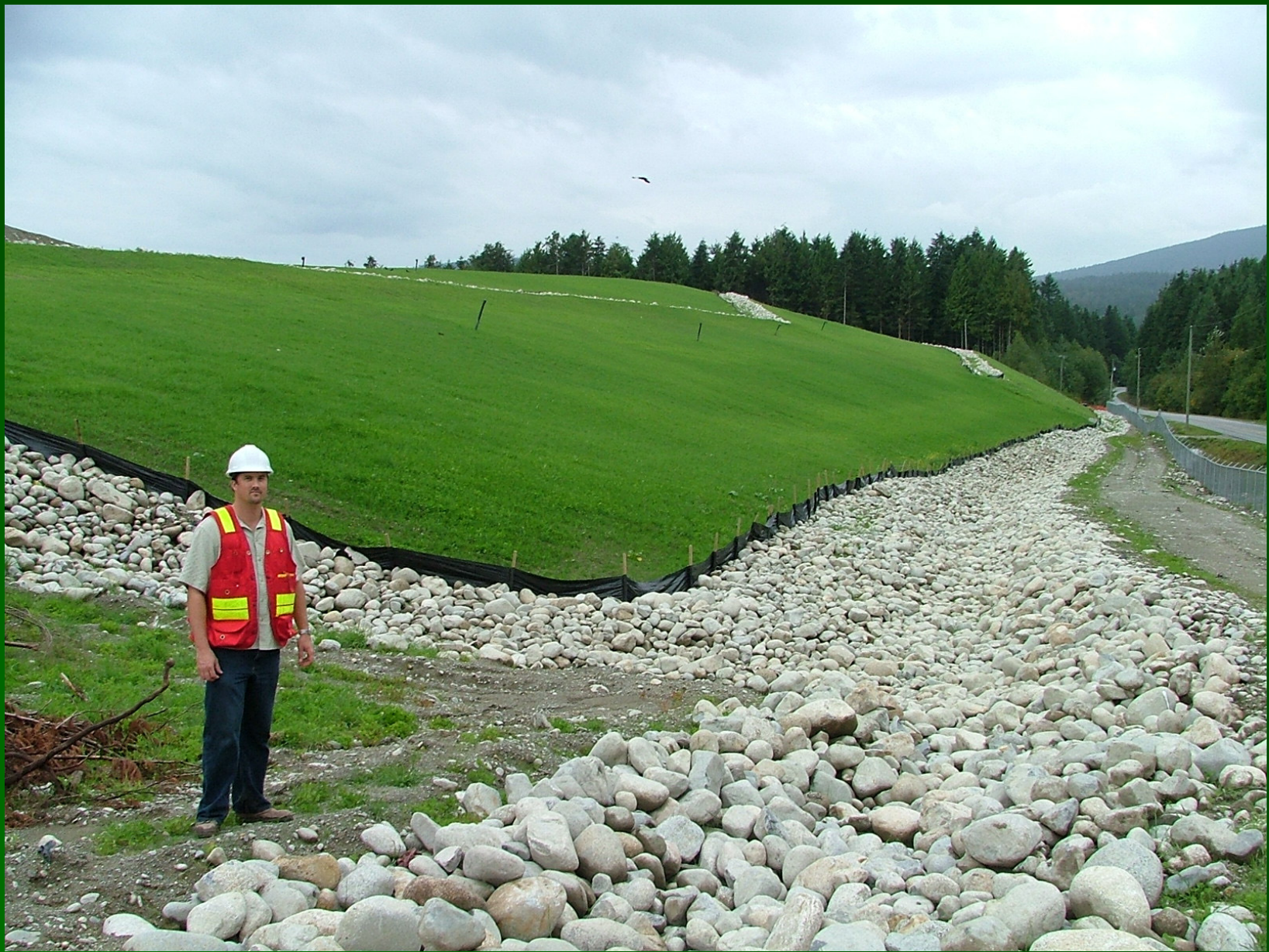
Geomembranes in Final Closure
