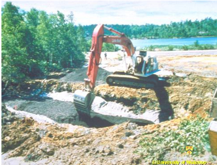
Sulfate reduction barrier, 1995
