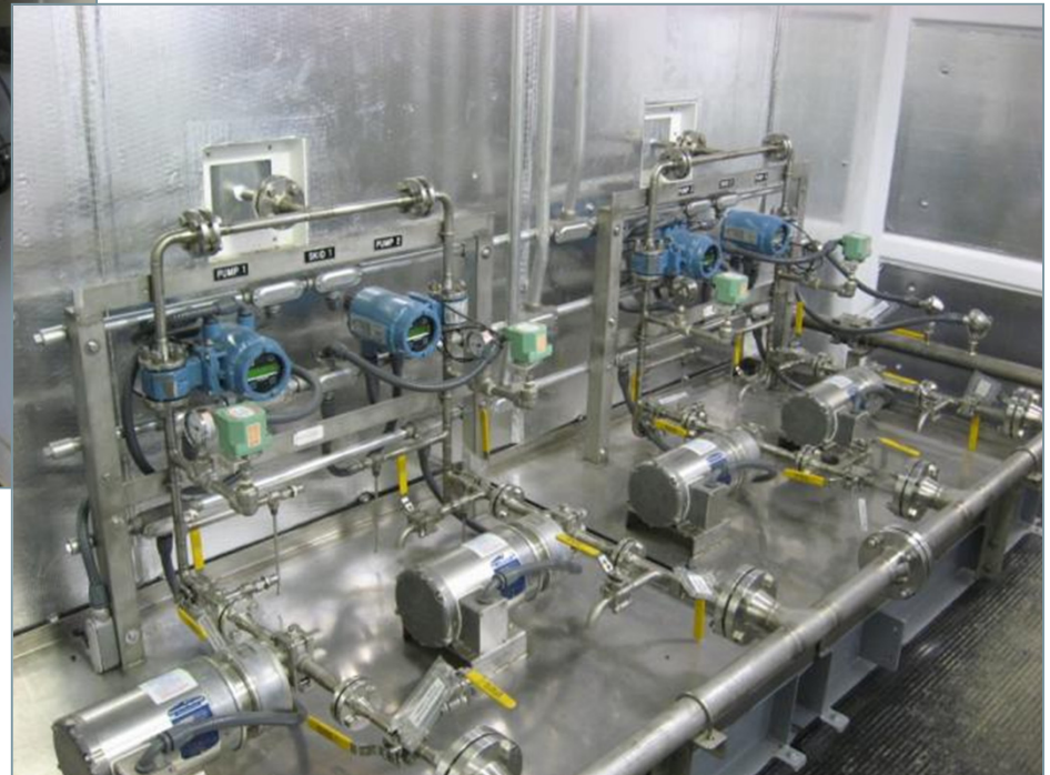
Hydrogen peroxide metering pumps (2 operating 2 spare)
