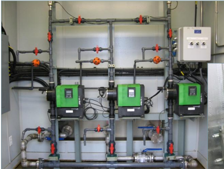
Ferric sulphate metering pumps (2 operating 1 spare)
