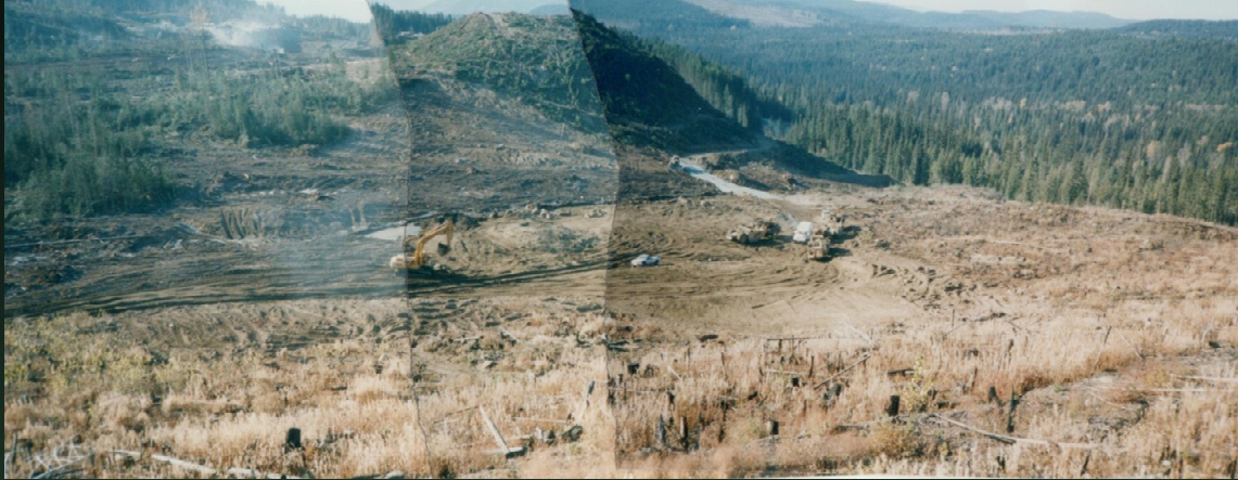
1988 view across impoundment, dam foundation started
