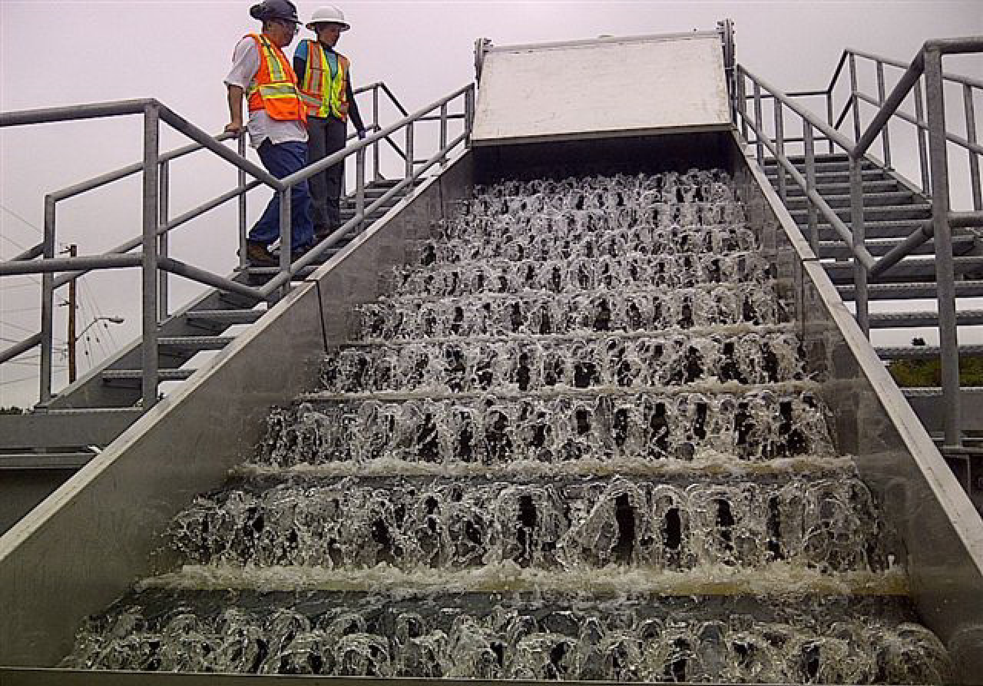
New Vic Aeration Cascades
