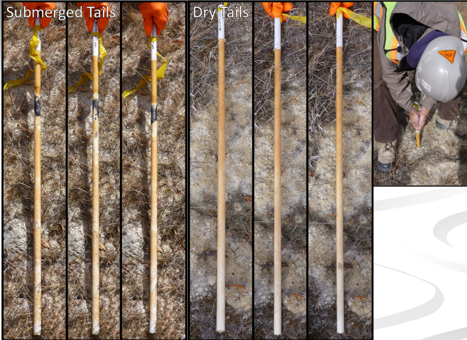
Photo 4.2-4: IRIS Tubes Installed in Water-Covered and Dry Tailings at Bethlehem Dam
