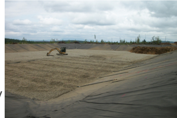
BCR Construction for sulfate removal in Canada (2012)
