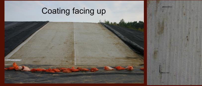
Upper GTX: Slit-film woven with impregnated polypropylene coating
