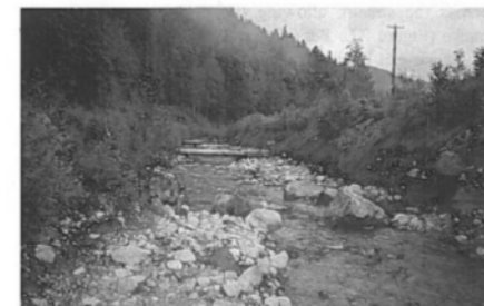
Figure 22. The Oulette Creek diversion channel four years after construction. The cross-vane rock sill in the foreground is buried in an infilled plunge pool. The 1.2-m diameter digger log in the background is undermined and suspended from the banks.
