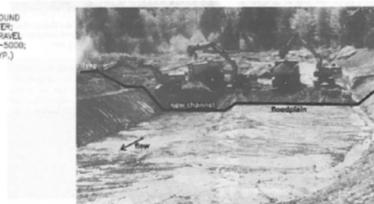
Figure 21. Construction of a 1.2-km long Oulette Creek diversion channel from the toe of the alluvial fan to Howe Sound, BC. Braided channels on the fan surface were installed for the development and protected by the dyke shown on the left. The design discharge at the constructed floodplain level was 17 m 3 /s.
