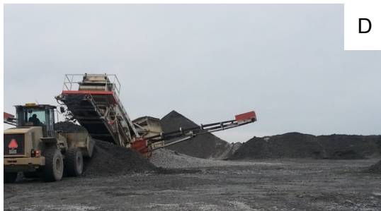
Carrying the paste rock to the storage area
