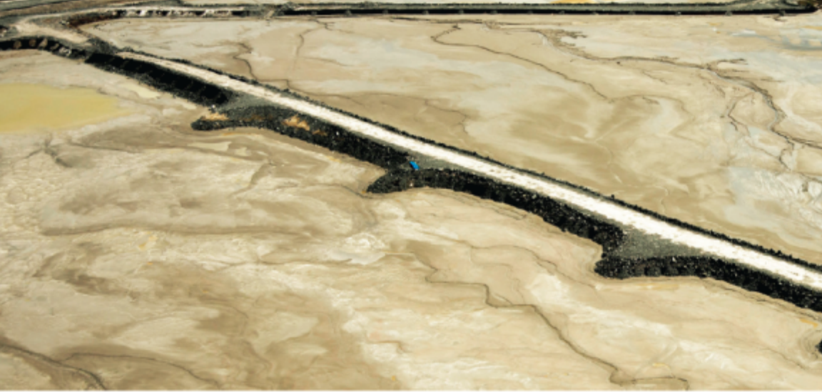
Waste rock inclusion constructed in the tailings impoundment at the Canadian Malartic mine. Such inclusions act as drainage and reinforcement elements to improve the hydro-geotechnical behaviour of the impoundment (photo provided by Osisko).
