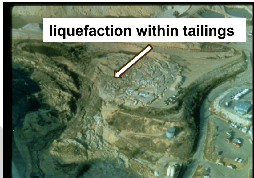
Tapo Canyon tailings impoundment USA, Northridge 1994 (adapted NISEE 2003)
