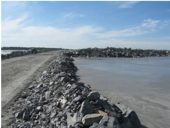
Figure 5. A waste rock inclusion in the tailings impoundment of the Canadian Malartic Mine (2016).
