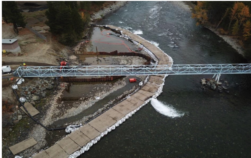
Overview of primary and secondary containment
