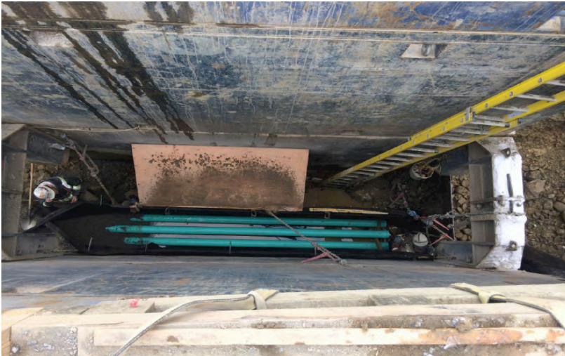
Collection piping installed in trench box, depths up to 8 m
