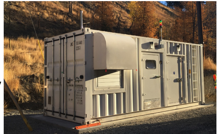
Back-up power generator housing
