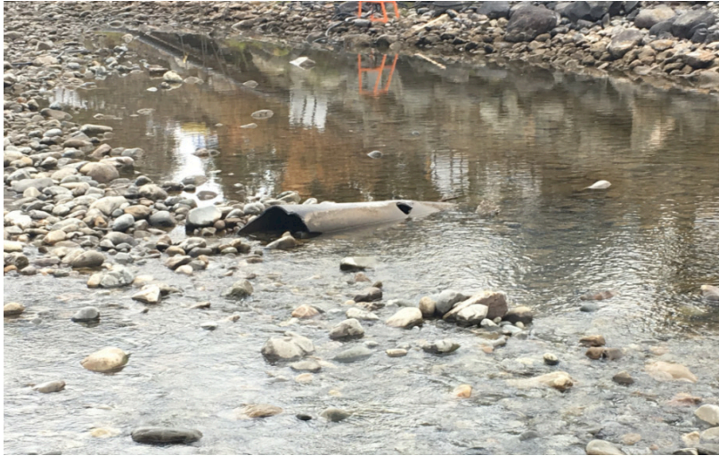
Damaged diffuser pipe
