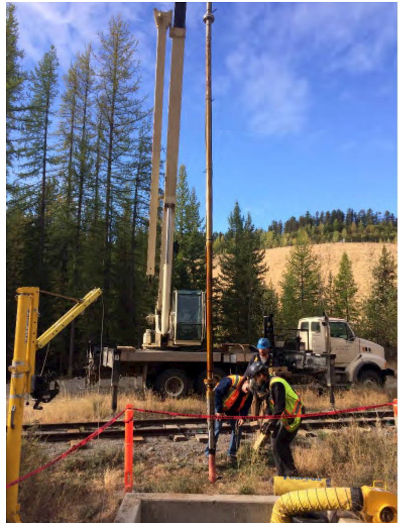
Pump removed from deep aquifer pump station for maintenance
