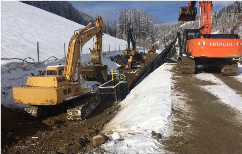
Interception trench excavation and collection system installation
