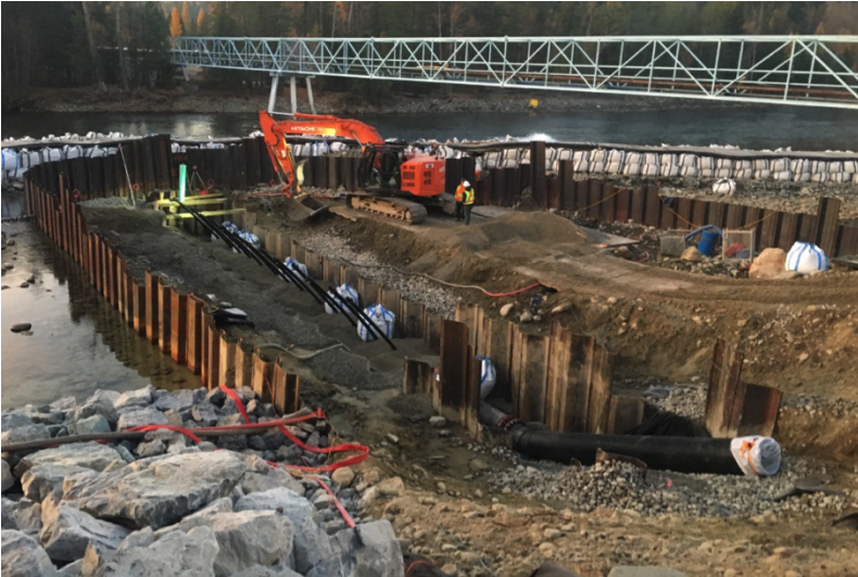
Diffuser pipe and riser installation
