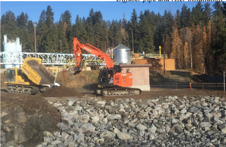
Site restoration above rip rap bank protection
