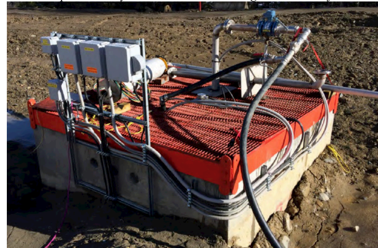
Collection vault, temporary pumping configuration
