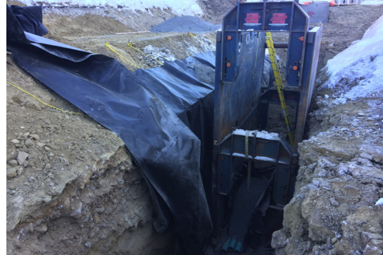
Low permeability liner installed on downgradient side of trench
