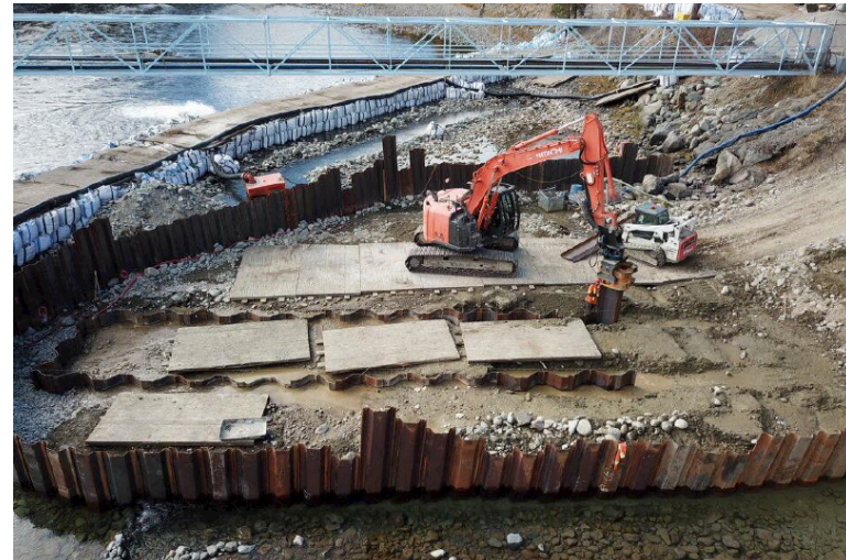
Installation of trench box with structural sheet pile
