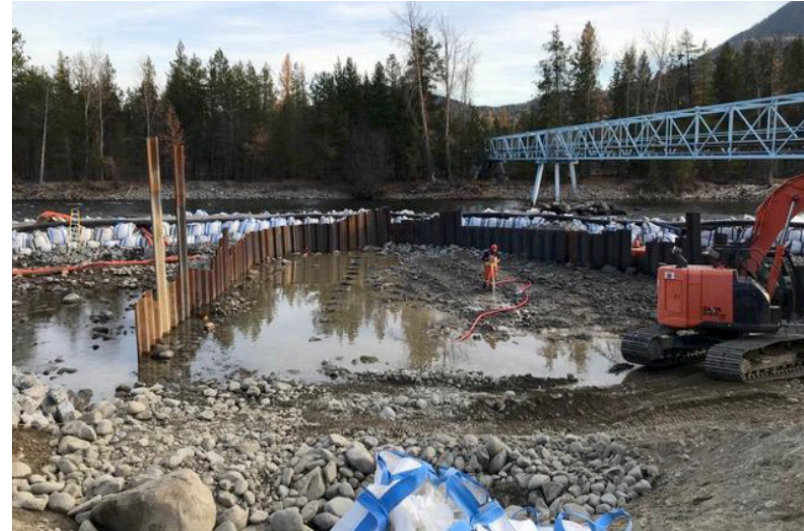
Sheet pile removal and bed restoration
