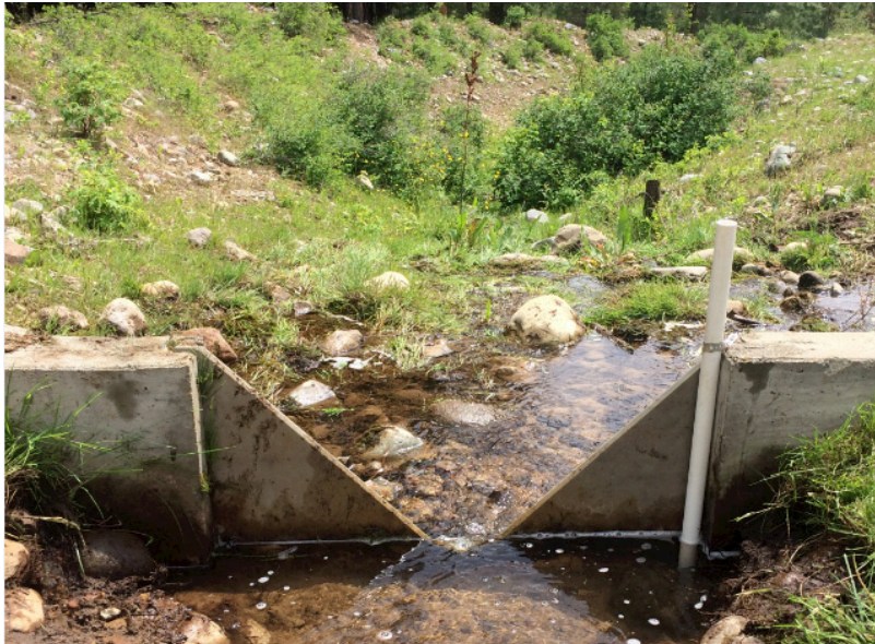
Weir at discharge point for Dobson's Draw diversion
