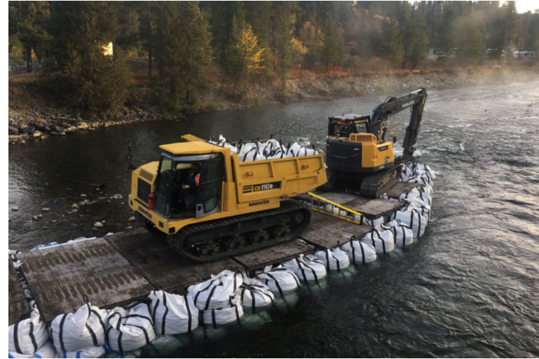
Construction of primary containment with gravel totes
