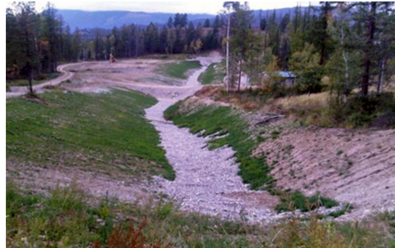
Backfilled groundwater interception trench system for PS937
