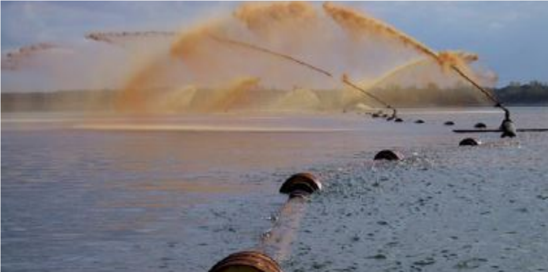
Addition of lime in Lake Koschen, Lusatian District, Germany (photo from Geller et al. 2012)
