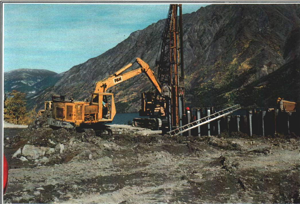
Photo 1: Waterloo Barrier Installation 5 September 1995
