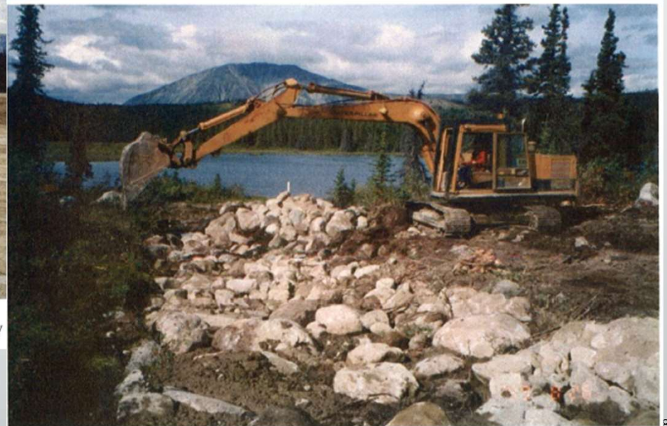
Photo 14 – Excavator placing riprap in drainage channel, August 1999.
