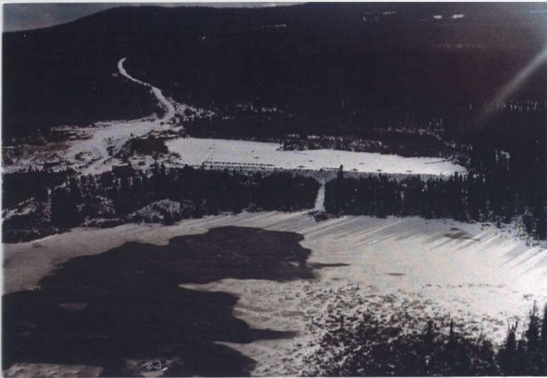
Photo# 1: Aerial View of the Tailings Impoundment and Drainage to Lake
