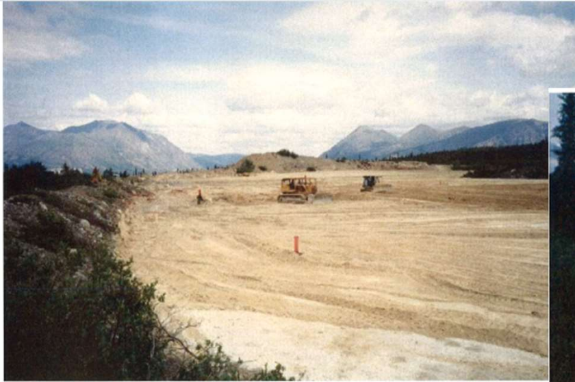
Photo 1 – Existing tailings impoundment being regraded by a D8 and D4 dozer, July
