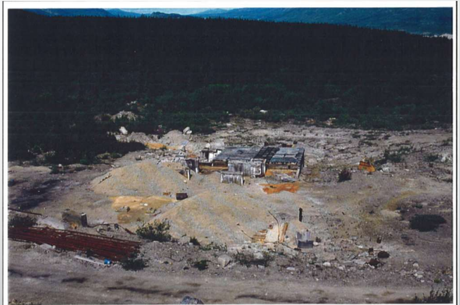
Photo# 11: Mill Site Foundation and Ore Piles
