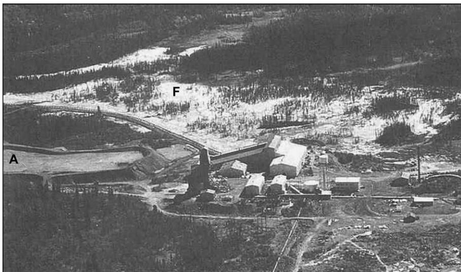
Fig. 2. The Nor-Acme Site, circa 1950. The Arsenopyrite Stockpile (A) was located north of the original mill, and the “emergency” flotation tailings (F) in a swamp to the east of the mill (Snow Lake Historical Records).
