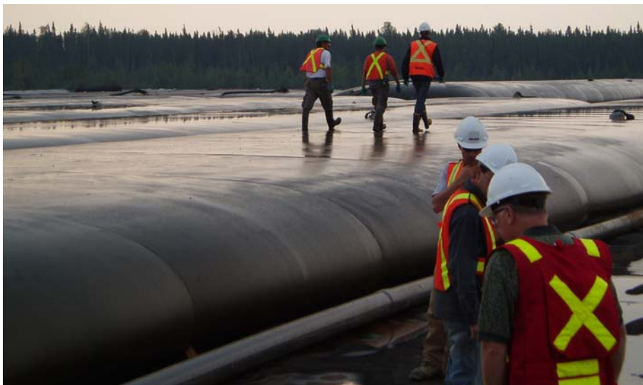
Fig. 7: The geotextile filter bags used for the temporary treatment of the contaminated pond water.
