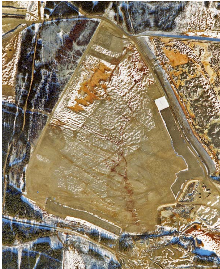
Fig. 7: Aerial view of the NIT area of the Kam Kotia Mine site during the construction of the remaining layers of the NIT cover. (Hazco - November, 2006).
