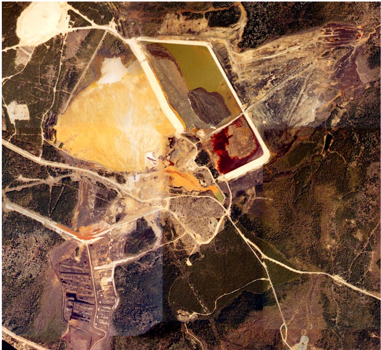
Fig. 5: Aerial view of the Kam Kotia Mine site after the completion of Phase “C” (May 2004).
