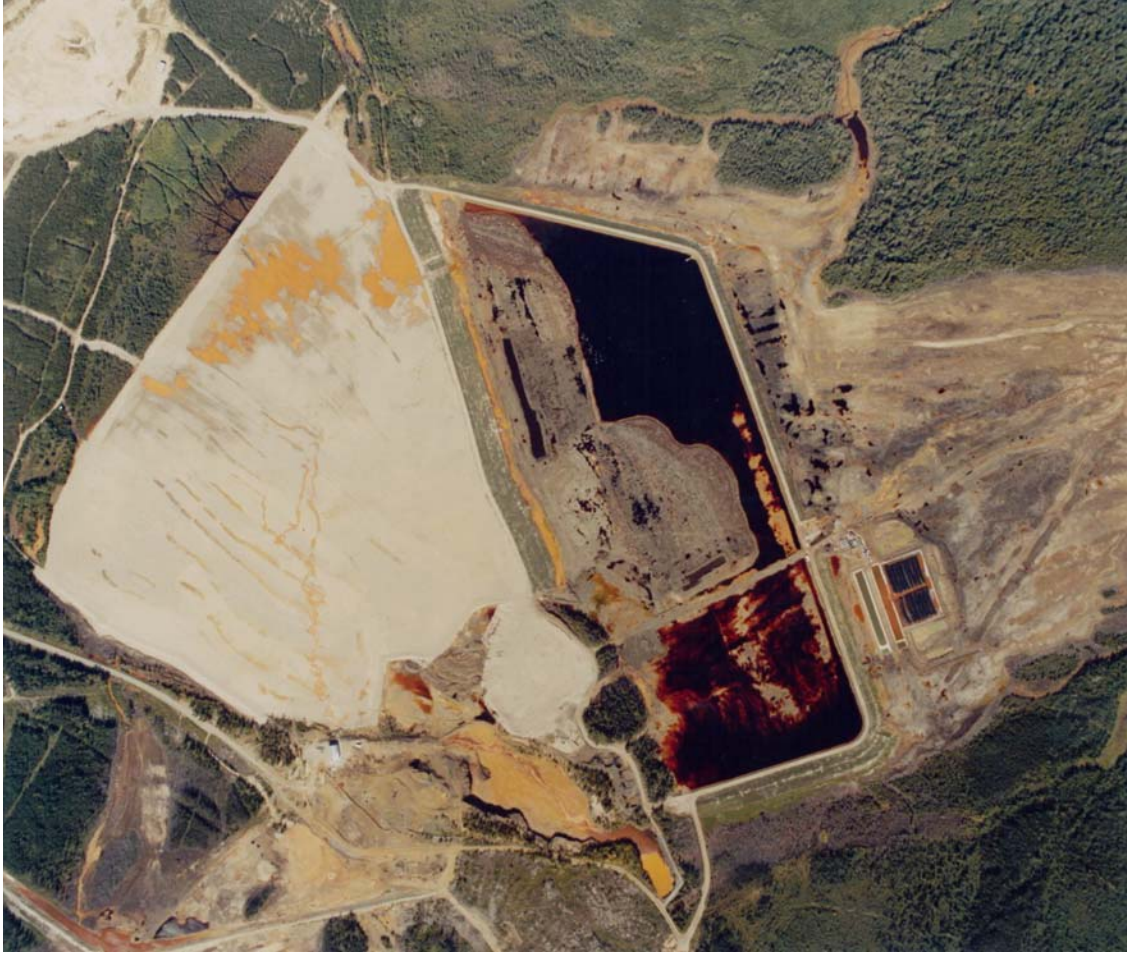
Fig. 6: Aerial view of the Kam Kotia Mine site after the construction of the NIT cover capillary break layers and the installation of the NUT area temporary water treatment plant near the southeast corner of the NUT impoundment dam (Hazco - June, 2005).
