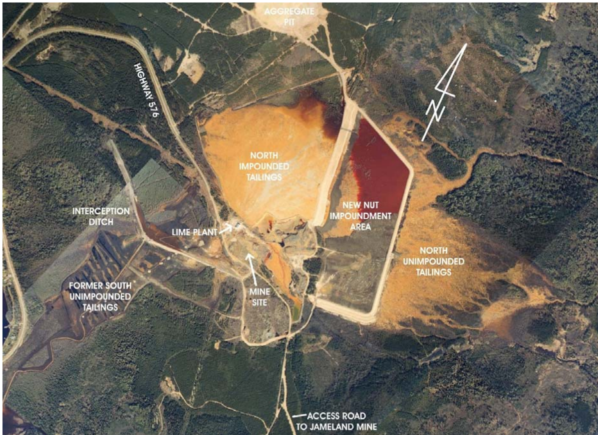
Fig. 4: Aerial view of the Kam Kotia Mine site after the completion of Phases “A” and “B” (May 2003).
