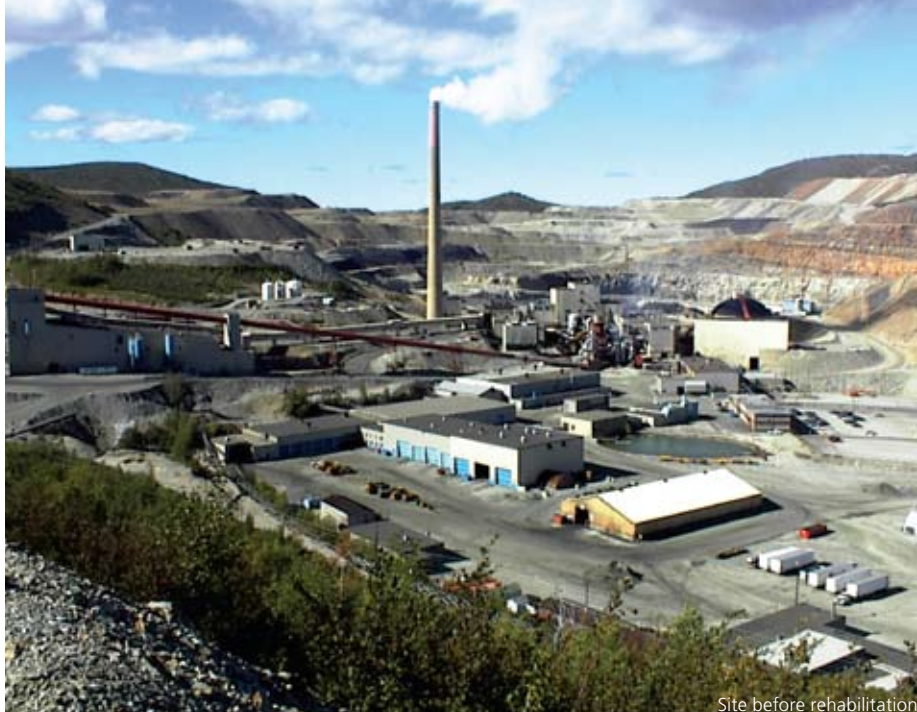
Site before rehabilitation
