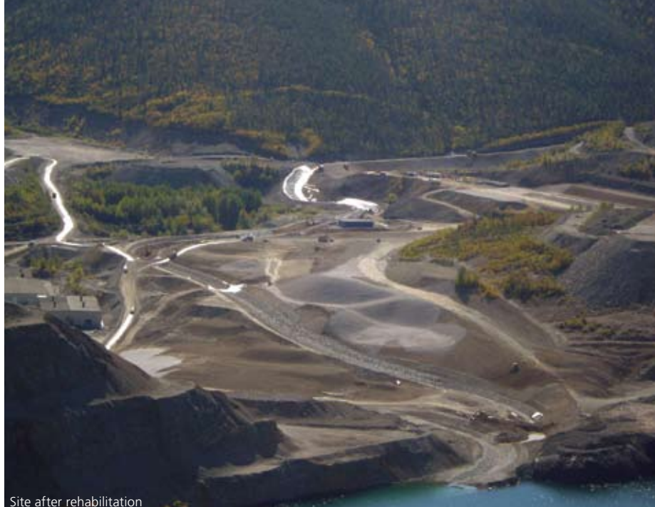
Site after rehabilitation
