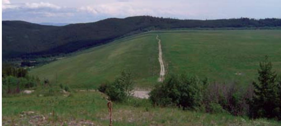
Main dam at Brenda Mines closed site
