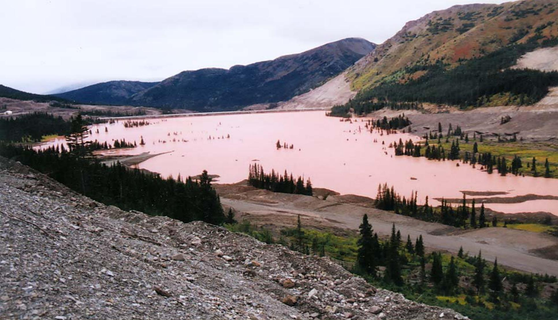
Except for a slight increase in Se, deposition of tailings from oxidized ore has had no adverse impact on impoundment water quality at Kemess.
