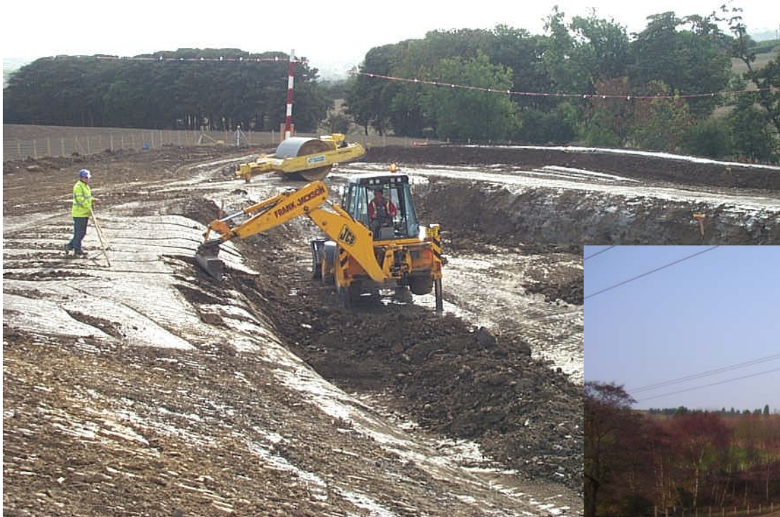
Construction (above) and completion (right) of Bowden Close RAPS system
