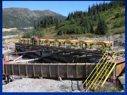
• 'Summer-only' flotation plant on long rougher tailings line. PAG concentrate sent to same place as old clnr-scav and short rougher tailings lines (underwater).
