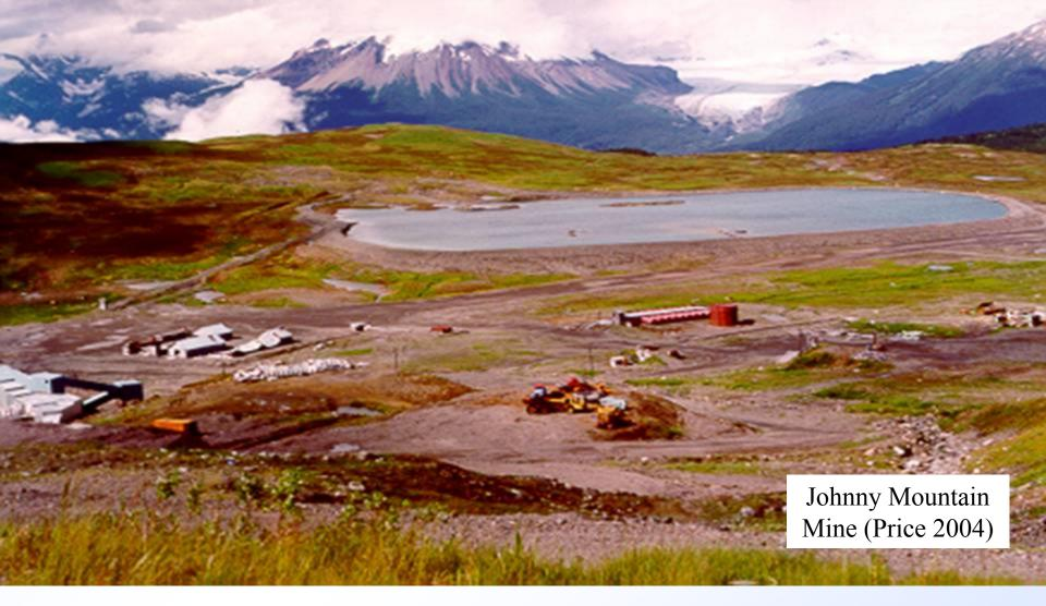
More dams are needed on flatter terrain away from water bodies. Dams were needed on three sides of the impoundment at Johnny Mountain. Use of mine wastes for dam construction reduces impoundment size and construction costs. At Huckleberry,
