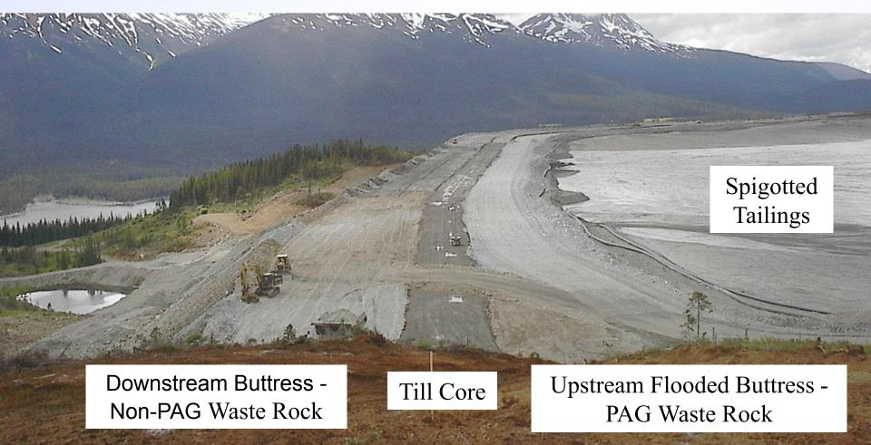
Dams are designed to withstand possible seismic and flood events. Buttresses are one way to increase seismic stability. The downstream buttress for the till core dam at Kemess South was constructed from desulphurized cyclone tailings sand (Bent 2008).
