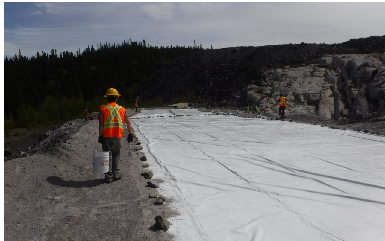
Installation of a plastic membrane (impermeable top-boundary)
