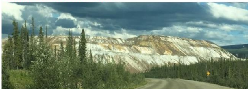
Evaporation causing formation of effluorescent salts
