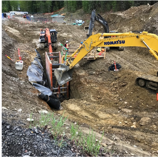
Pull access shoring cage access to next section, 60T machine
