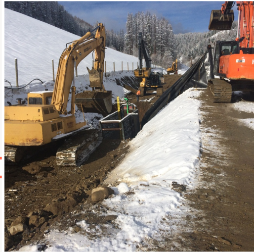
Pre-excavation of trench, depths 6 m to 7 m, for shoring cage access, 15 m 'segments'
