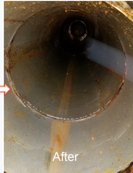
3900 Mine Line After Jet Rod and Pipe Pig
