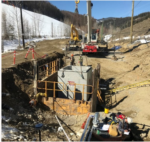
North Trench Upgrade Vault Installation
