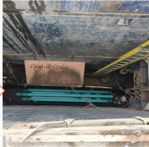
Place perforate pipes, pea gravel, geotextile wrap,
