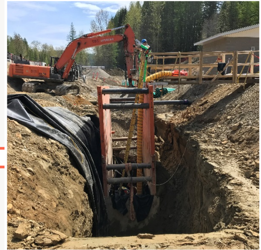
Install liner outside access shoring cage, and set up for pipe fusing
