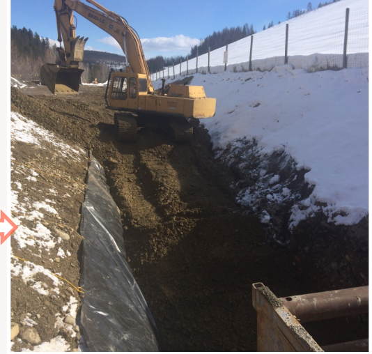
Backfill and compaction, excavated soil from next section
