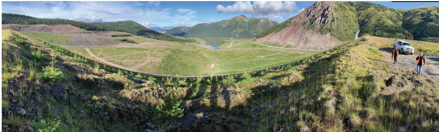
Kemess South TSF embankment
