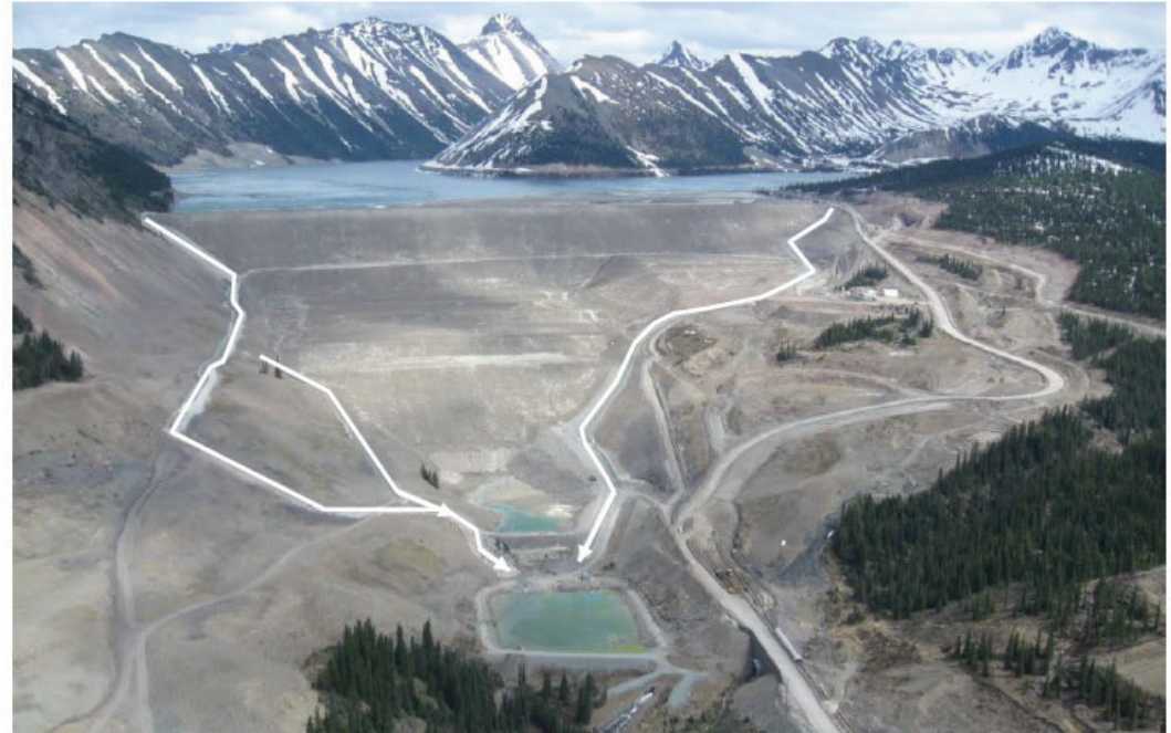
Figure 3.8: Runoff Diversion Ditches (white arrows). Photo taken May 2010.
