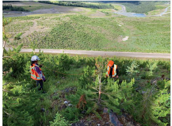
Kemes South TSF embankment looking South
