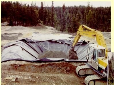
CCBE: sand, over tailings or silt, over sand, over reactive tailings
