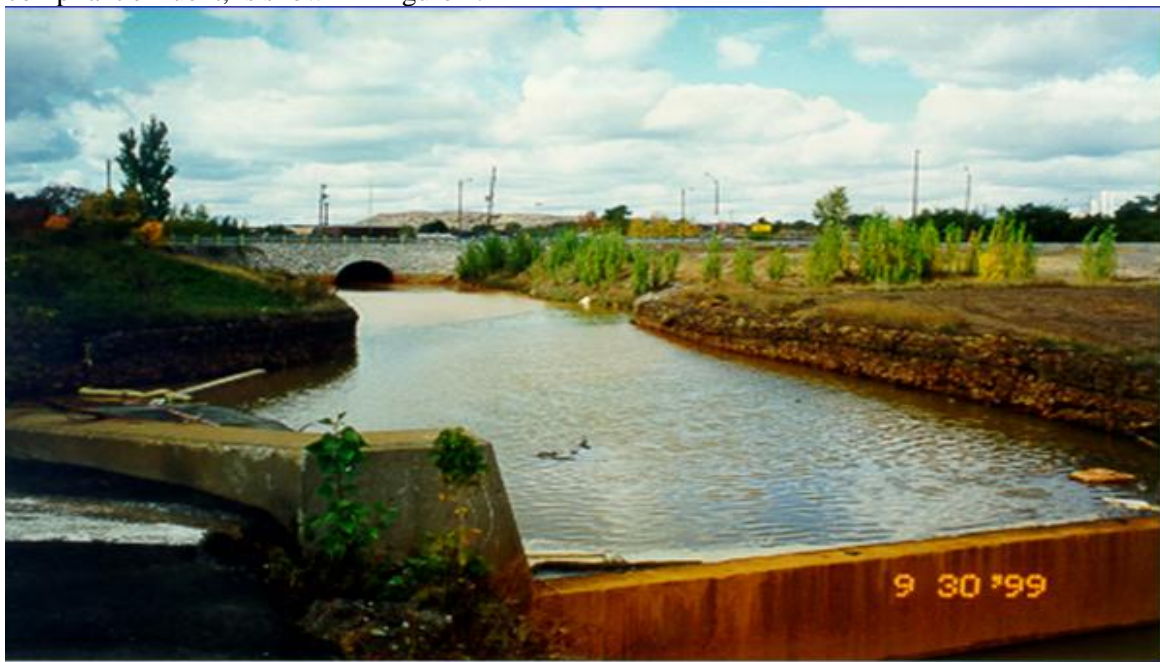
Figure 2: Copper Cliff Creek looking upstream through the CCWWTP Bypass Weir.
