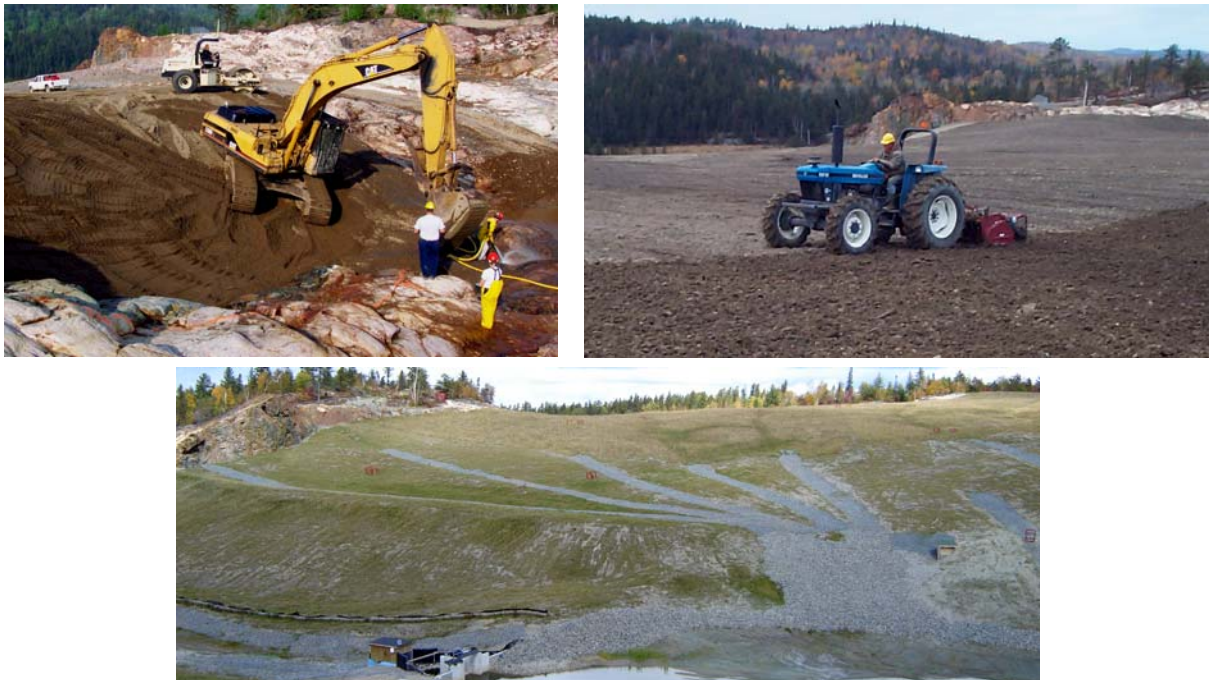
Figure 4 Photos showing cleaning of the pit perimeter prior to barrier layer construction (top left), cross-slope ripping of topsoil into the granular cover material (top right), and the finished pit cover in Sept-06 with the Collection Pond overshoot gate in the foreground (bottom)
