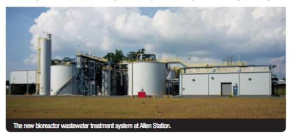
activated carbon for the microbes to attach to and grow on, nutrient or "food" source for the organisms and specifications for the biological system. The construction consortium provided the process and mechanical design for the biological system and built the concrete biological reactors.
